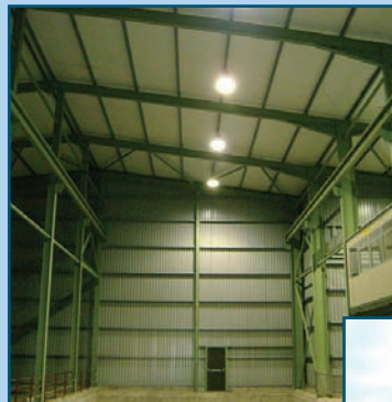
Shed 2 portable frame building internal
